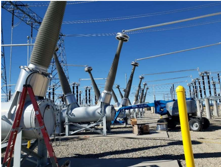
Figure 8. Breaker bushings
