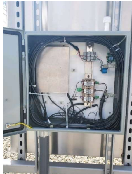
Figure 12. Another vendor cabinet with fiber cables installed in the yard
