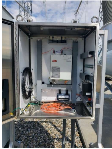
Figure 11 One vendor cabinet with FOCUS electronics module installed in the yard
