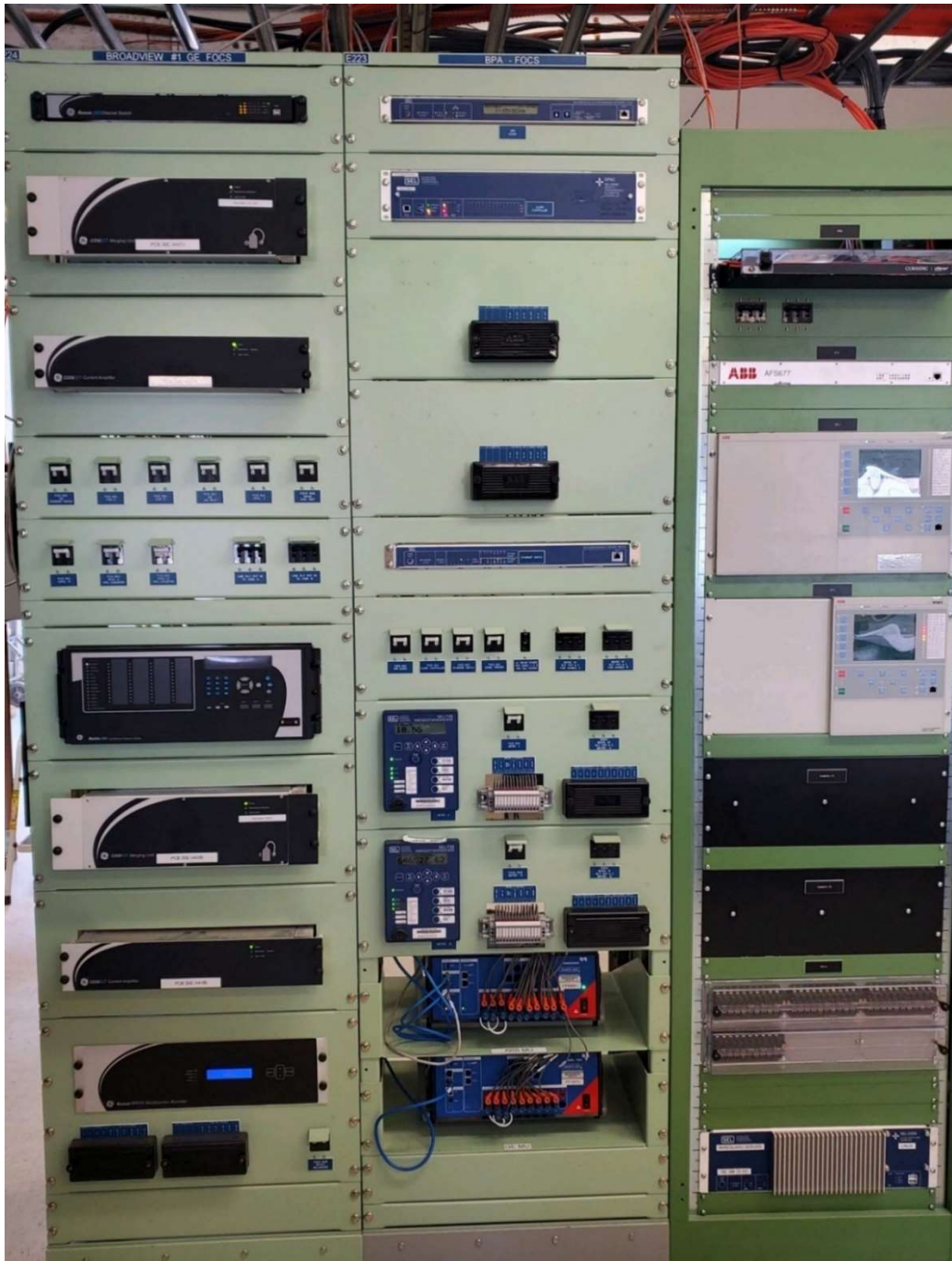
Figure 13. Three panels installed in the control house
