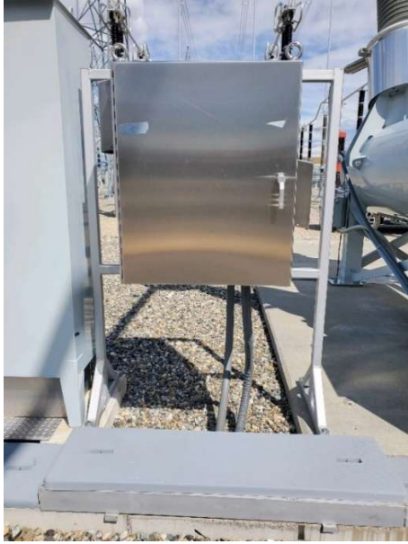
Figure 11 One vendor cabinet with FOCUS electronics module installed in the yard
