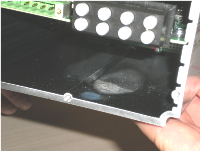
Fig. 26. With CT Board Removed, Heat and Arc Damage Evident
