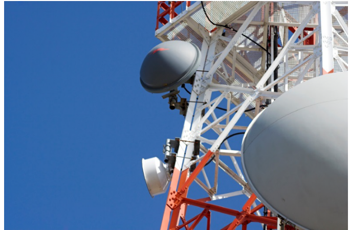
Fig. 9. Microwave dish antenna and tower
