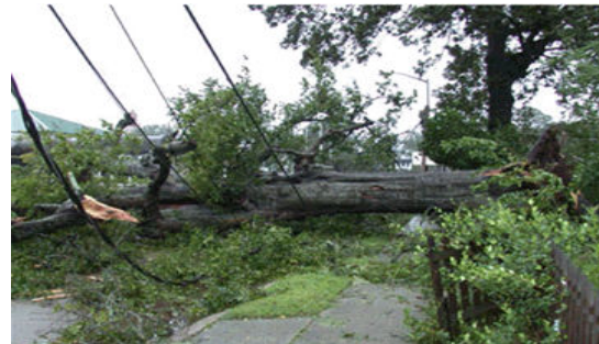
Fig. 1. Downed conductors
