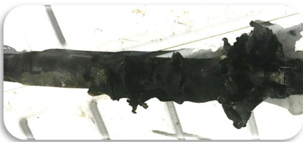
Figure 16 Cable splice which failed during staged fault testing
