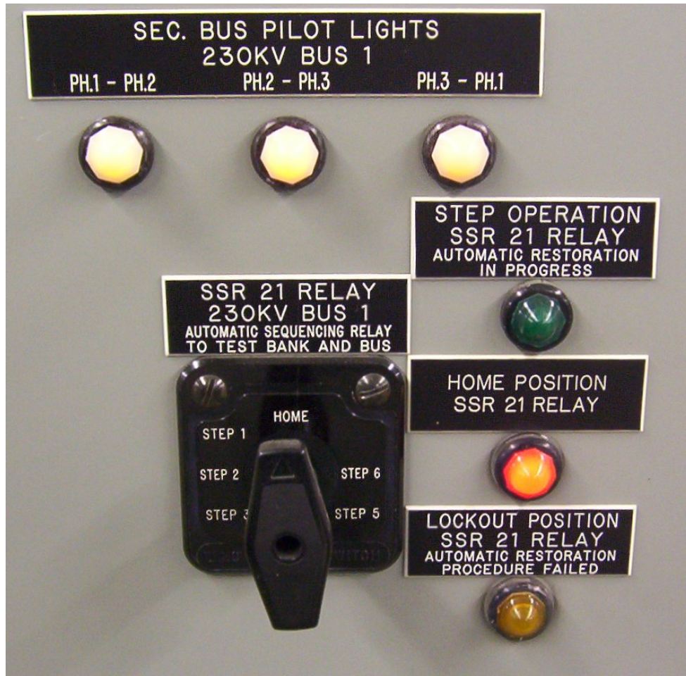
Figure 7 - Close up of stepper switch showing indicator lights for reset (home), in-progress and lockout
