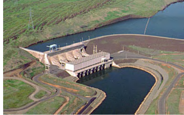
Fig. 2. Thermalito Power Plant
