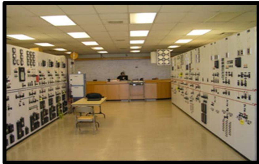
Figure 6 – Spacious former center aisle in P&C building.
