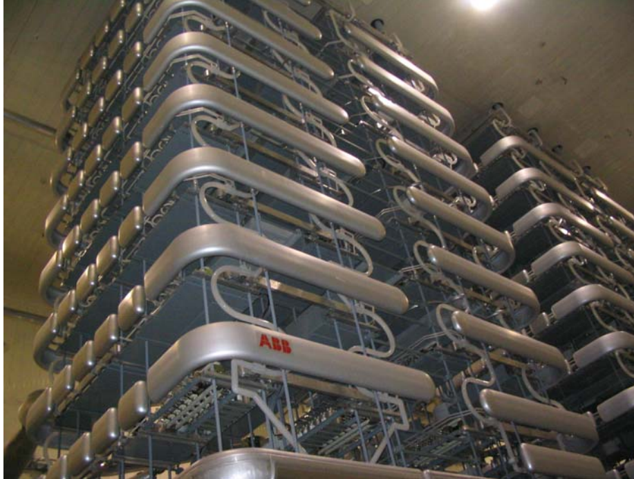
Figure 3. New Bi-pole installation at LADWP.
