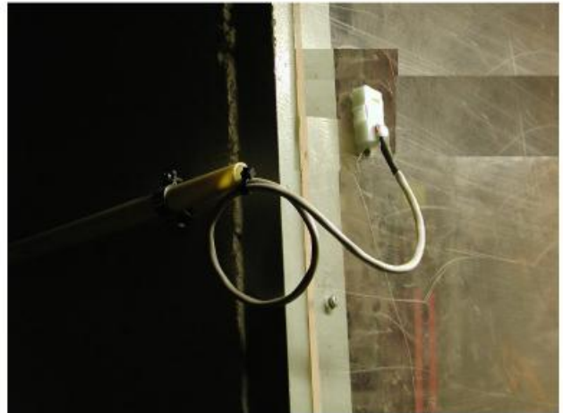
Figure 11. An Arc sensor installed at wall of a cubicle.
