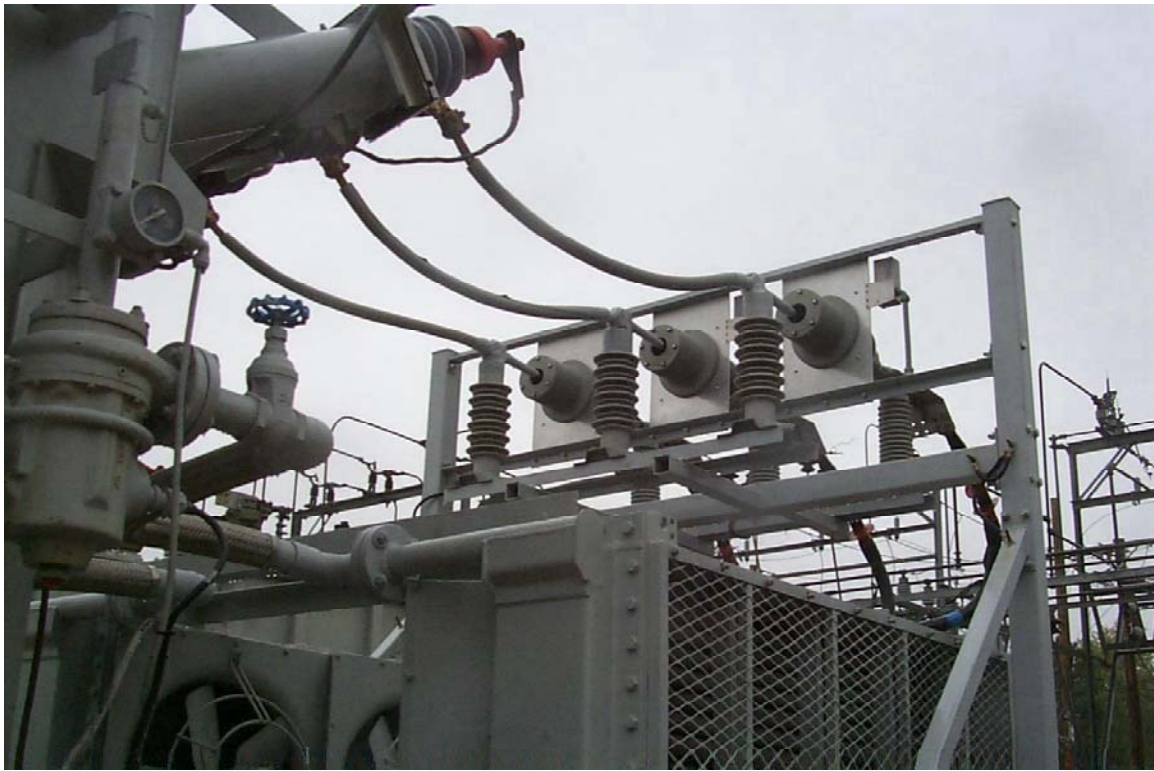
Figure 24. Secondary Side Rogowski Coils
