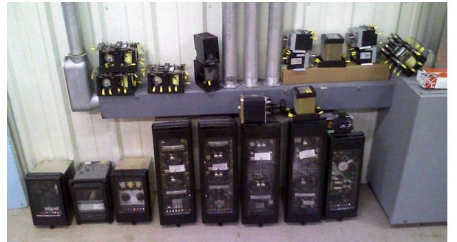
Fig. 2. Electromechanical distance scheme components.
