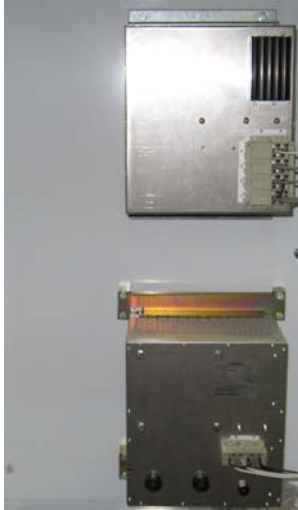
Figure 1: 20 Hz Generator and Bandpass Filter
