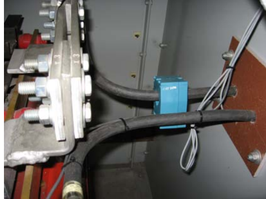
Figure 2: Miniature CT to measure 20 Hz current
