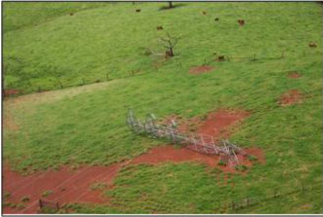
Fig. 47. Collapsed tower as a result of Cyclone Larry (category 5 wind speed)—GW was broken at one location
